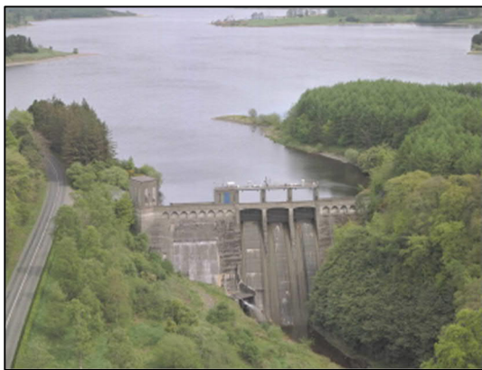
Figure 2. Poulaphouca Dam & Reservoir
